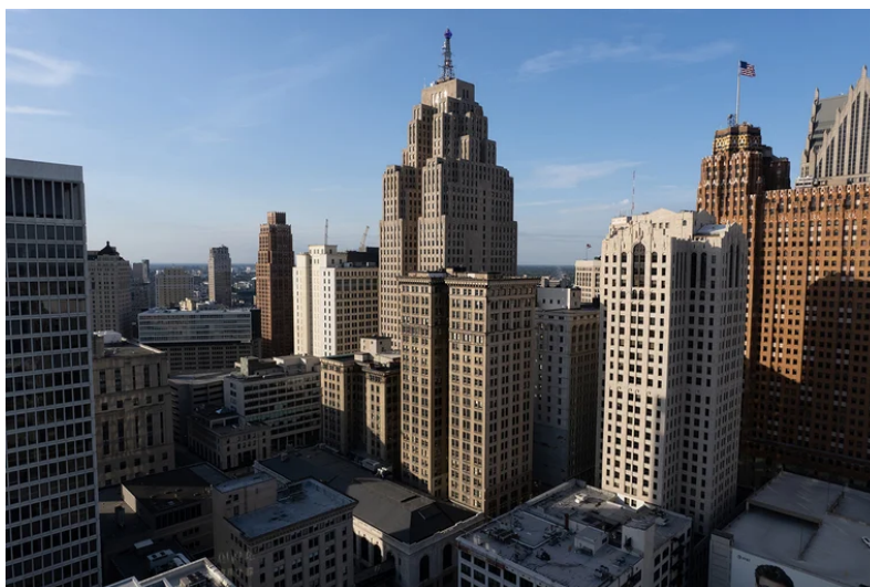
The Penobscot Building downtown has a new brokerage firm marketing it for lease.
